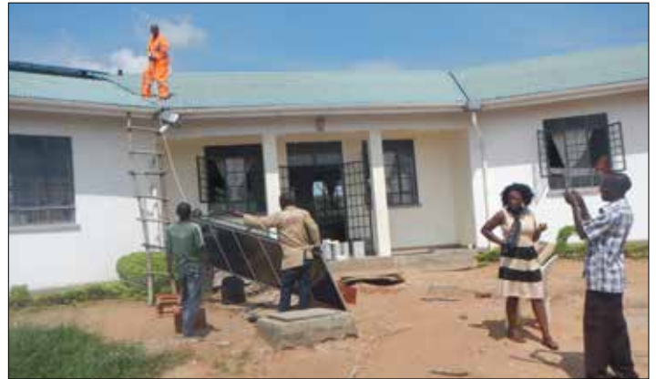
Left: Assembling solar panels in their frames before installing them on the roof top. Right: Installing solar panels on the roof of a Blue House Building. Chairman of the Uganda Board of Blue House and Matron Agnes were present for the installation of the panels.
