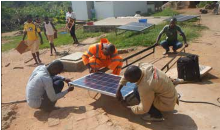
Left: Assembling solar panels in their frames before installing them on the roof top. Right: Installing solar panels on the roof of a Blue House Building. Chairman of the Uganda Board of Blue House and Matron Agnes were present for the installation of the panels.
